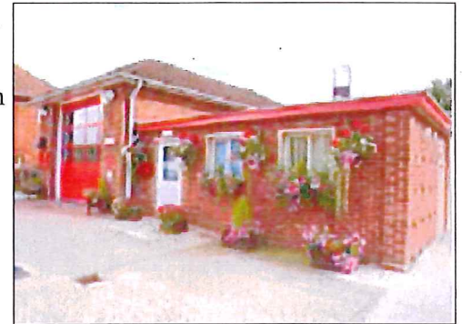
Brinklow Fire station—Heath Lane
